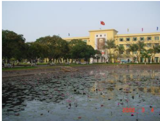
The HUA's Administrative Building where CARES is located
